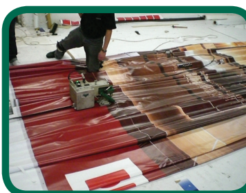
Track Welding on Floor
